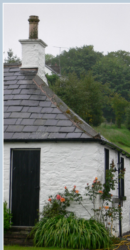
Regular courses, but random widths of local slate fixed using a double-lap method under stone ridge pieces. Dumfries & Galloway.
