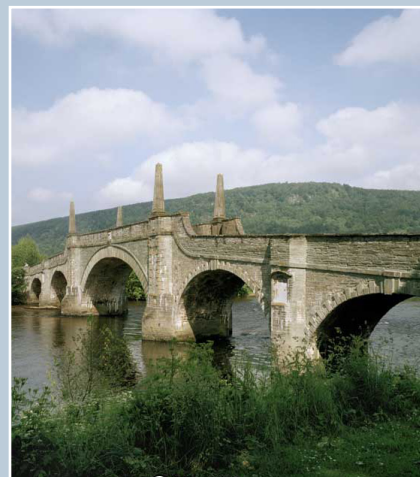
Aberfeldy Bridge, Perth & Kinross, showpiece of General Wade's military road network, combines cutwaters with neo-classical quoins and obelisks that signal the springing point of the arch. © Crown copyright: RCAHMS. Licensor www.rcahms.gov.uk .
