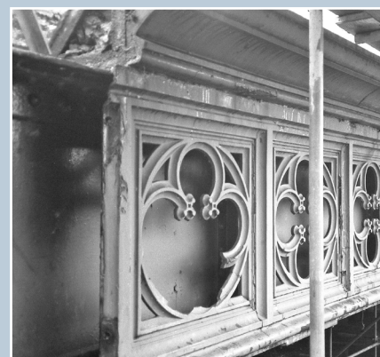
Dalmarnock Bridge, Glasgow, is a series of wrought iron girders behind a gothic cast-iron panel. It was strengthened in 1996 by insertion of new steelwork. The repaired cast-iron parapet is protected from traffic by bollards.
