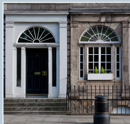
The old conversion of the right-hand doorway to a window and removal of the main entrance steps is disruptive to the character of the building and the broader pattern of entrances and windows in the street. © N. Haynes.
