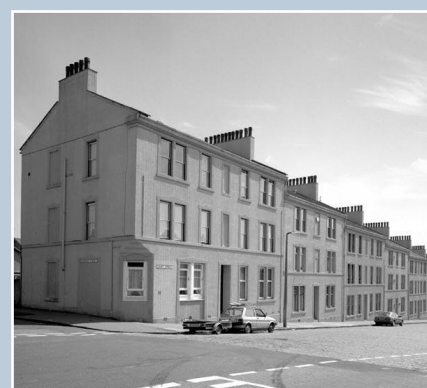
Mass concrete tenements in Dundee, cast insitu in 1874–5 by the Concrete Building Company for the Working Men's House Building Association. The buildings were renovated and a buff render applied in 1982–4. © Crown copyright: RCAHMS. Licensors www.rcahms.gov.uk .
