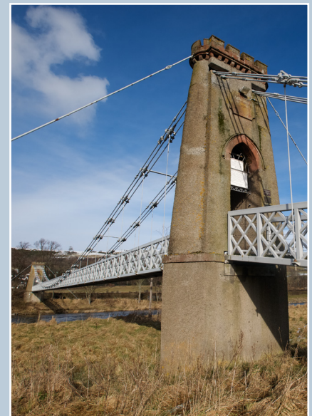
The same bridge at Gattonside after its reconstruction in 1991–2. The parapet of the same bridge is so straight that it now acts as a girder. Chains and connections are much heavier and while some fabric has been retained its character is compromised.
