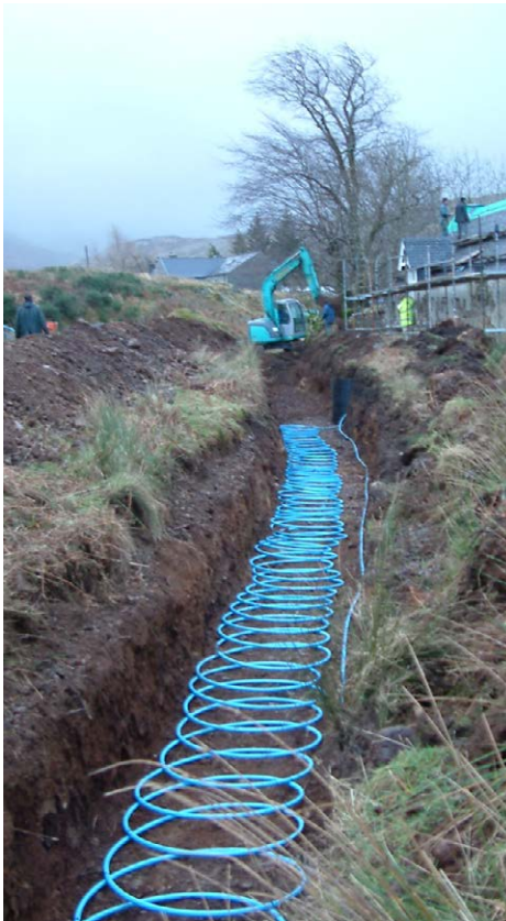
Installation of a ground-source heat pump (GSHP) at Assynt Church, Inchnadamph (Category B-listed). The coils for the system were installed in trenches behind the church. © LDN Architects
